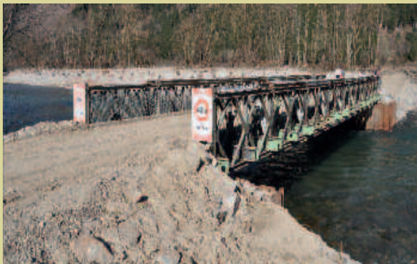
Provisional bridge. A temporary bridge was built over the Drau between January and April 2011 to help with the construction work on the right bank of the river.
