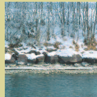
Problem: Due to increased river bed erosion, the riverbank control structures become unstable and threaten to collapse. Simultaneously, the groundwater level sinks. A problem for the wetlands, agriculture and flood protection.
