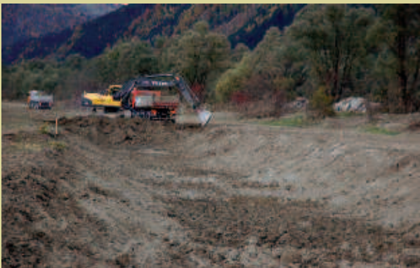
Mass movement. During the river widening at Obergottesfeld, a total of 200.000 m 3 of soil and gravel were moved.
